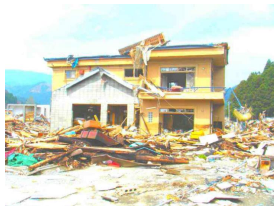
Figure 8 Totally inundated house by the Great East Japan Earthquake and Tsunami 2011. The tsunami height was higher than the roof judging from debris on the roof. CHB wall structure got almost no damage. (Source: Hiroko Minoda and Yasumichi Mifune)
