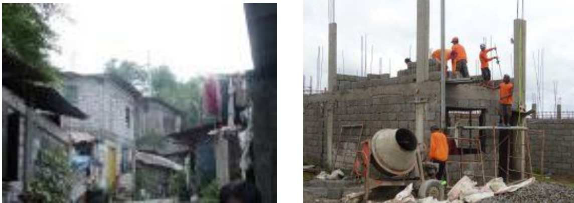
Figure 1 CHB houses in the Philippines. Left: residential area of low/middle income people in Payatas, Metro Manila, Right: construction for middle income people by a developer, Metro Manila
