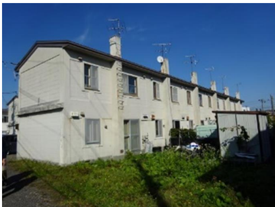
Figure 7 Rental CHB houses by municipal government of Eniwa City, Hokkaido. Still in use after about 50 years since construction.
