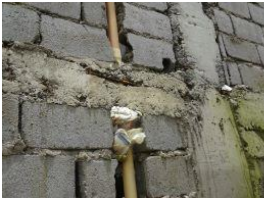
Figure 4 Construction site by a developer. Left: construction work of CHB wall with pipe for electric cable, Right: Appearance becomes pretty good after finishing work
