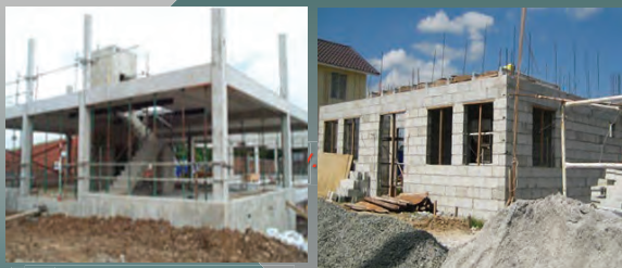
Conventional Portal Frame Construction System
