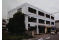
Completed in 1987 Gunma Block Kaikan Reinforced CHB construction 3 stories
