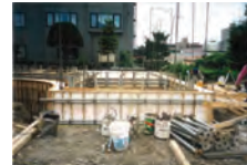
Formwork for foundation
