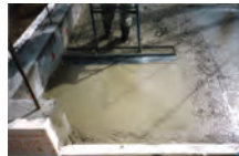
Leveling concrete
