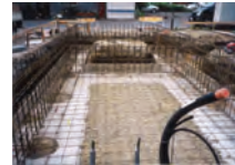
Placement of rebar for foundation
