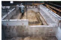
Leveling concrete
