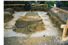
Formwork for foundation
