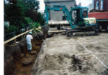
Placement of rebar for foundation
