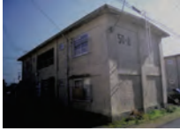
1950 Gunma Prefectural Housing (A block made from coal waste is used as a curtain wall)
