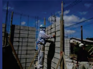
It takes time to lay CHB units and grout mortar.
