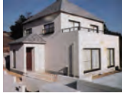
"House 30" model house Formwork block construction
