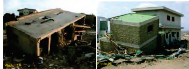
⑤ Over-turning due to tsunami ⑥ Inclination due to uneven ground settlement Heavy damages were not found on upper structure.
