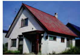
Government financed housing with quasi-fire-resistant structure (Triangular roof type reinforced CHB structure)
