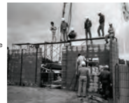
Floor height filling situation of filling mortar
