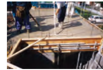
Leveling concrete on the second floor
